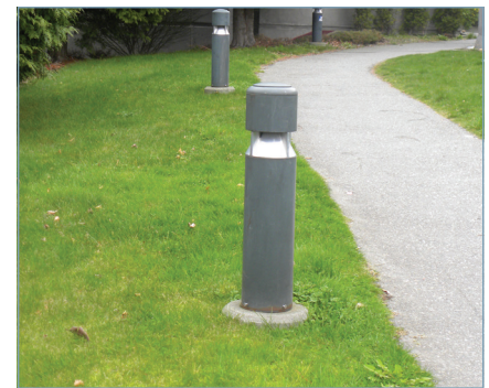
2.5.2.h.ii Standard illuminated bollard.
