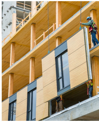
Images of UBC Brock Commons tall wood student residence with pannelized construction.
