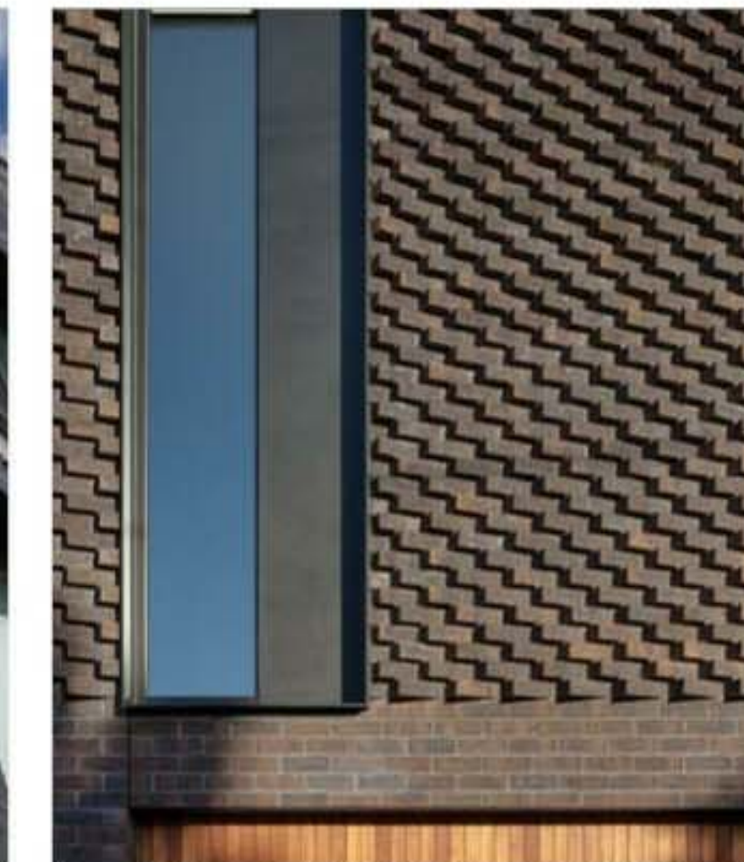
Balwyn North - Matyas Architects
