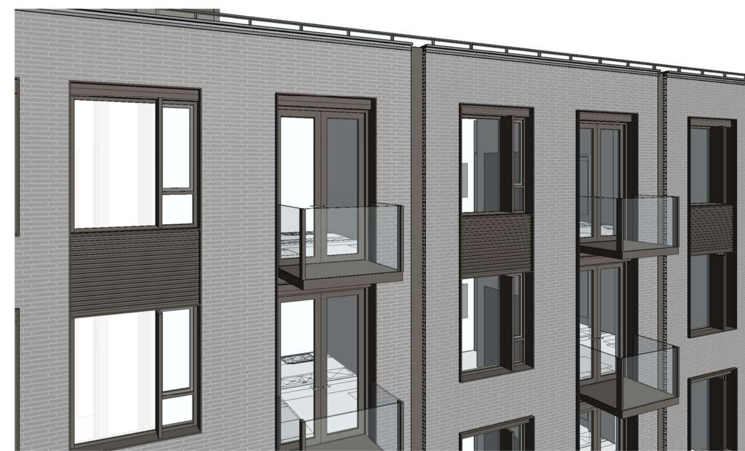
2 VIEW OF BALCONIES
