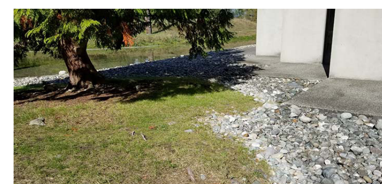
View G13 Sheet L4 (G13:L4) existing site conditions | roots of cedar visible in foreground of photo - meters outside of tree dripline | critical root zone must be protected during construction activities
