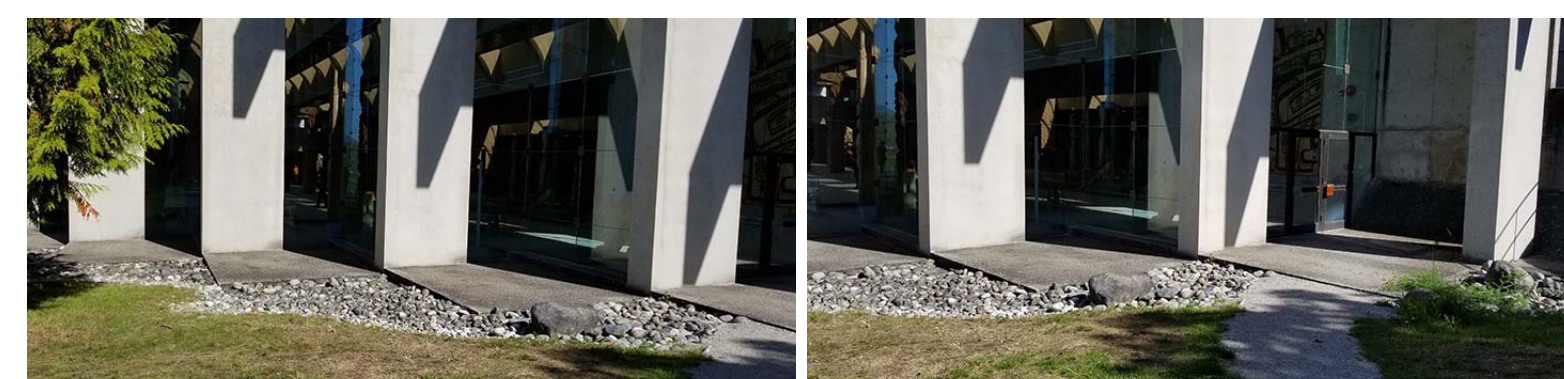
Views G14 Sheet L4 (G14:L4) existing site conditions | vegetation | aggregate concrete pads | cobbles | path | site elements
