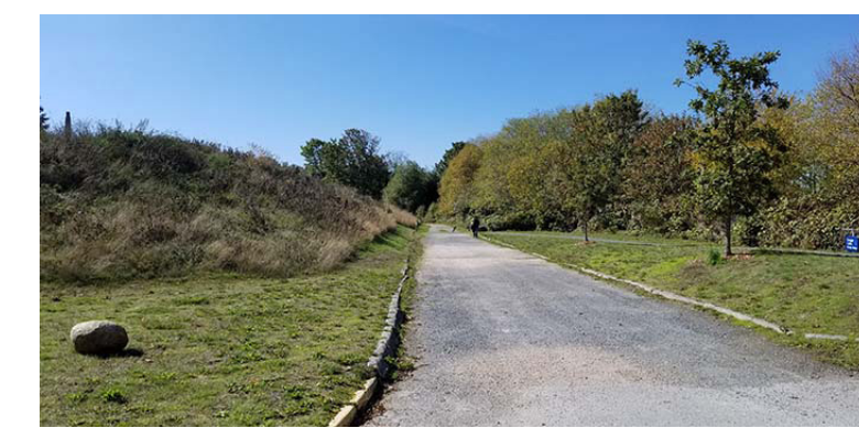
View G28 Sheet L5 (G28:L5) existing site conditions | proposed location of temporary vehicle access route | vegetation | grading | path | oaks require critical root zone protection fencing
