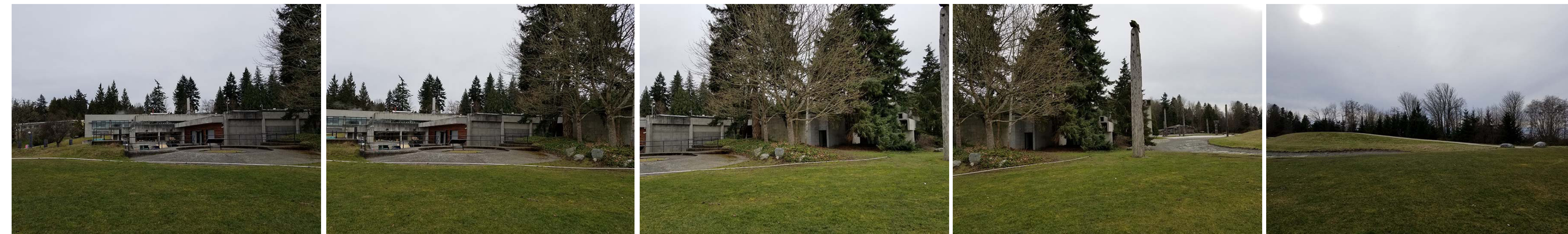
Views G35 Sheet L4 (G35:L4) existing site conditions | armory / gun emplacement | totem | vegetation | hemlock | cobbles | grading | views toward area proposed for construction set-up and staging and temporary construction vehicle access route on mound, west edge of pond
