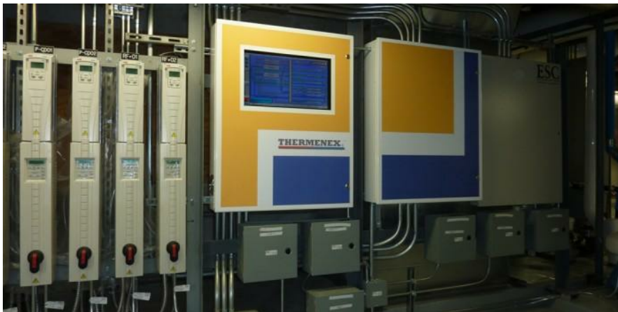
existing thermonex heating and cooling system with monitoring and controls
