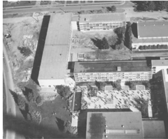
West Courtyard with East Courtyard under construction, 1960
