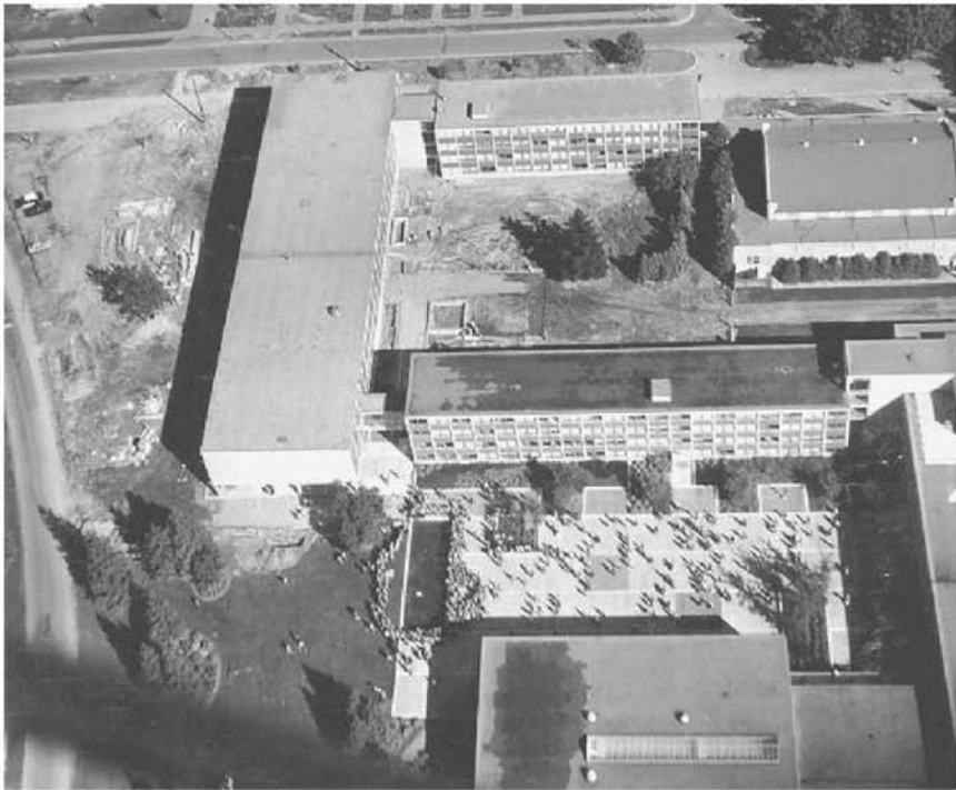
West Courtyard with East Courtyard under construction, 1960
