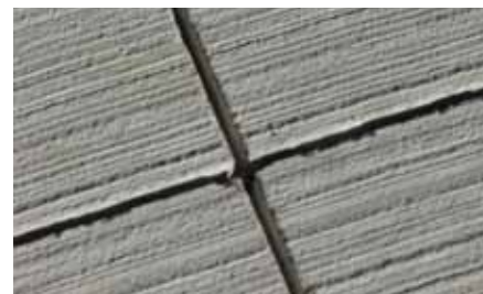
Saw Cut Concrete Paving
