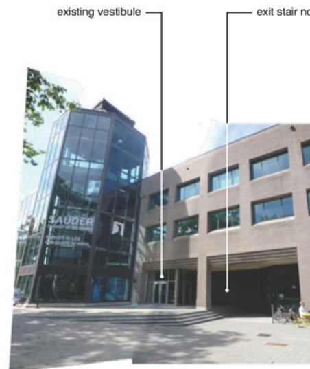
4 Existing Entrance looking West
