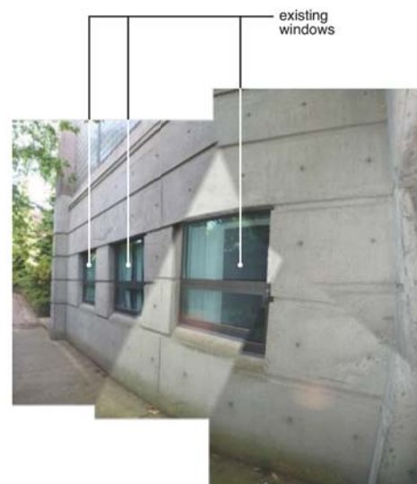
4 Existing External Wall
