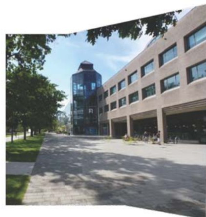
3 Existing Entrance looking South
