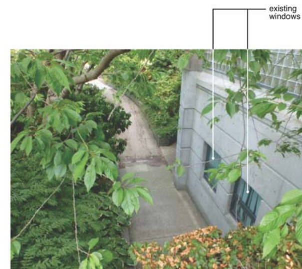
5 Existing Access Path from above
