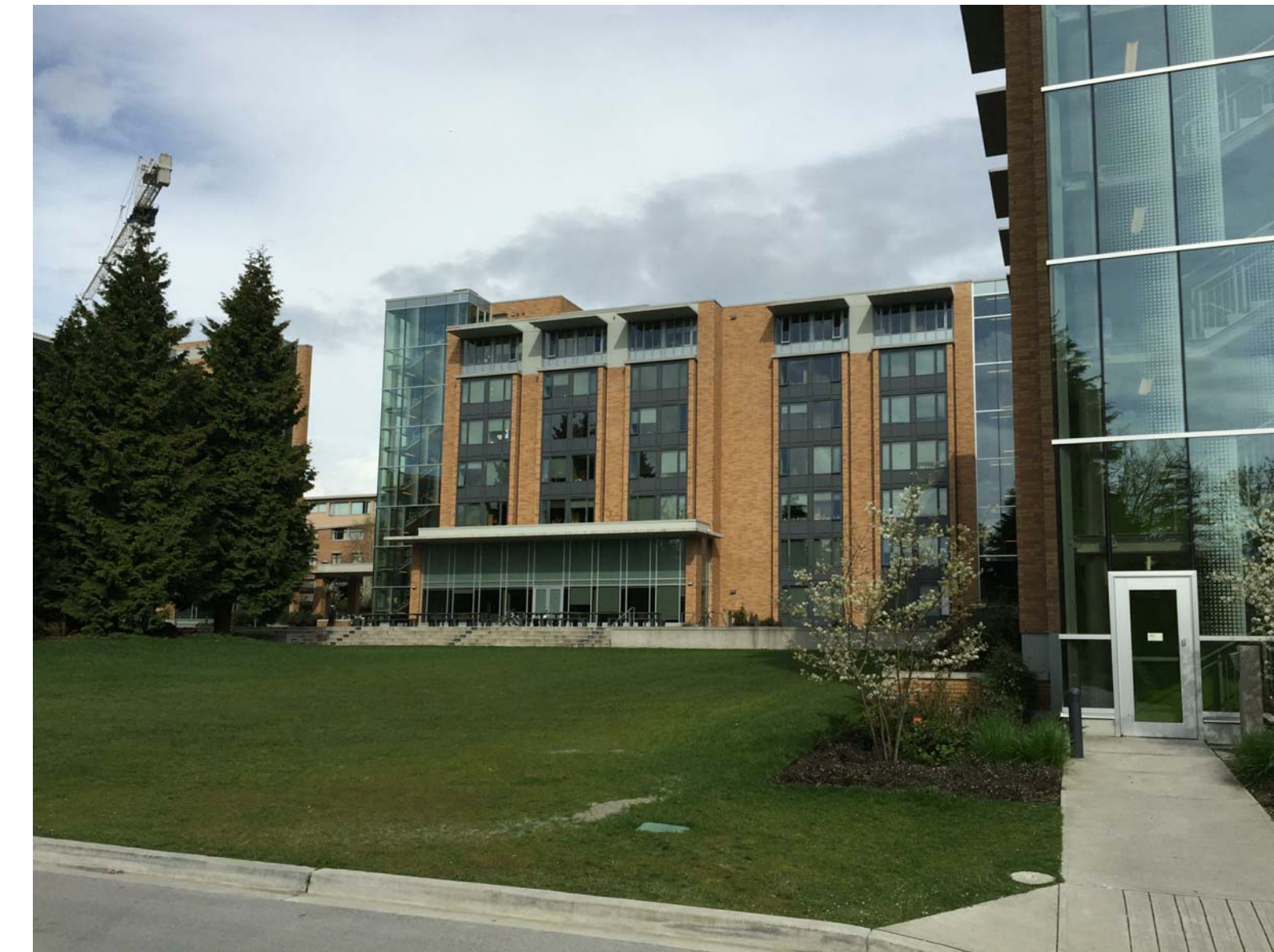
Looking east at Hemlesem House
