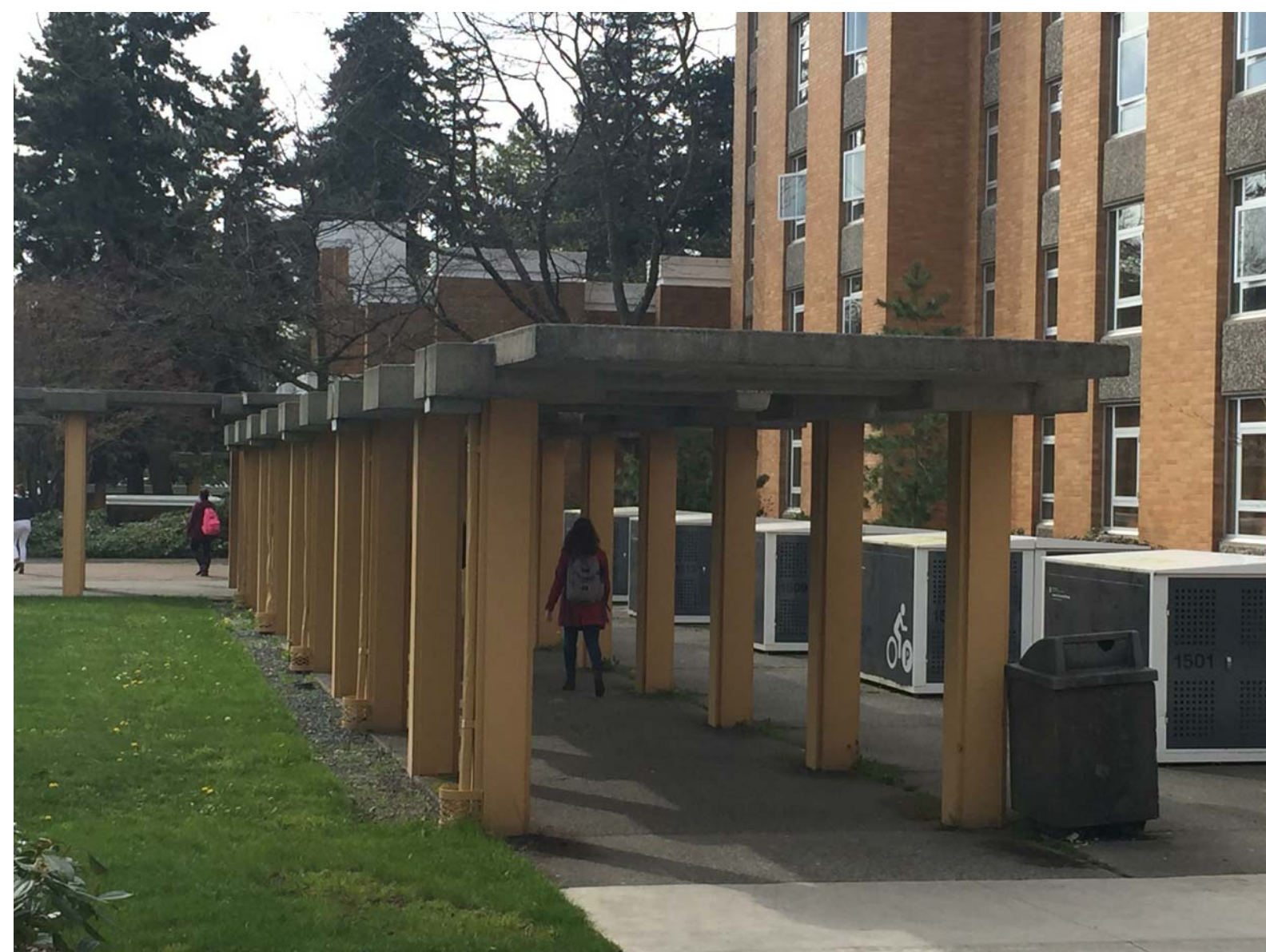
Totem Park rain protection network
