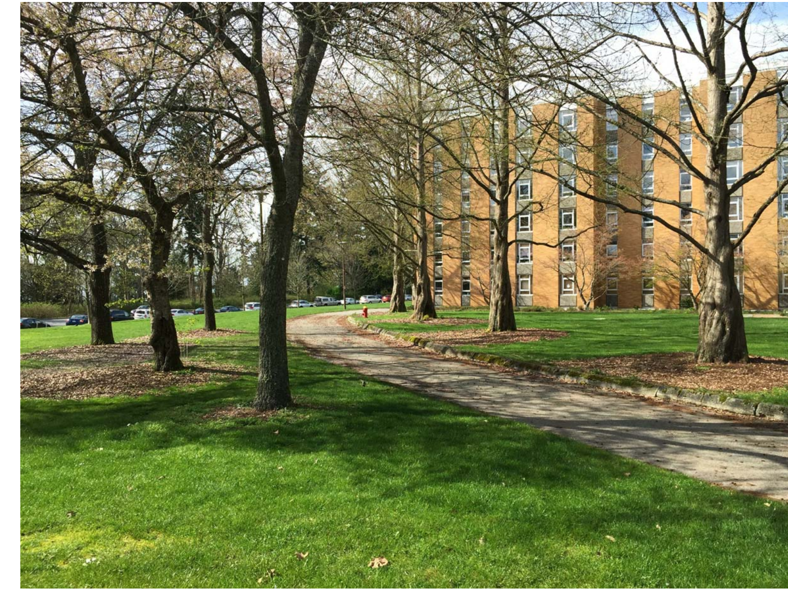
Looking west along existing fire access road
