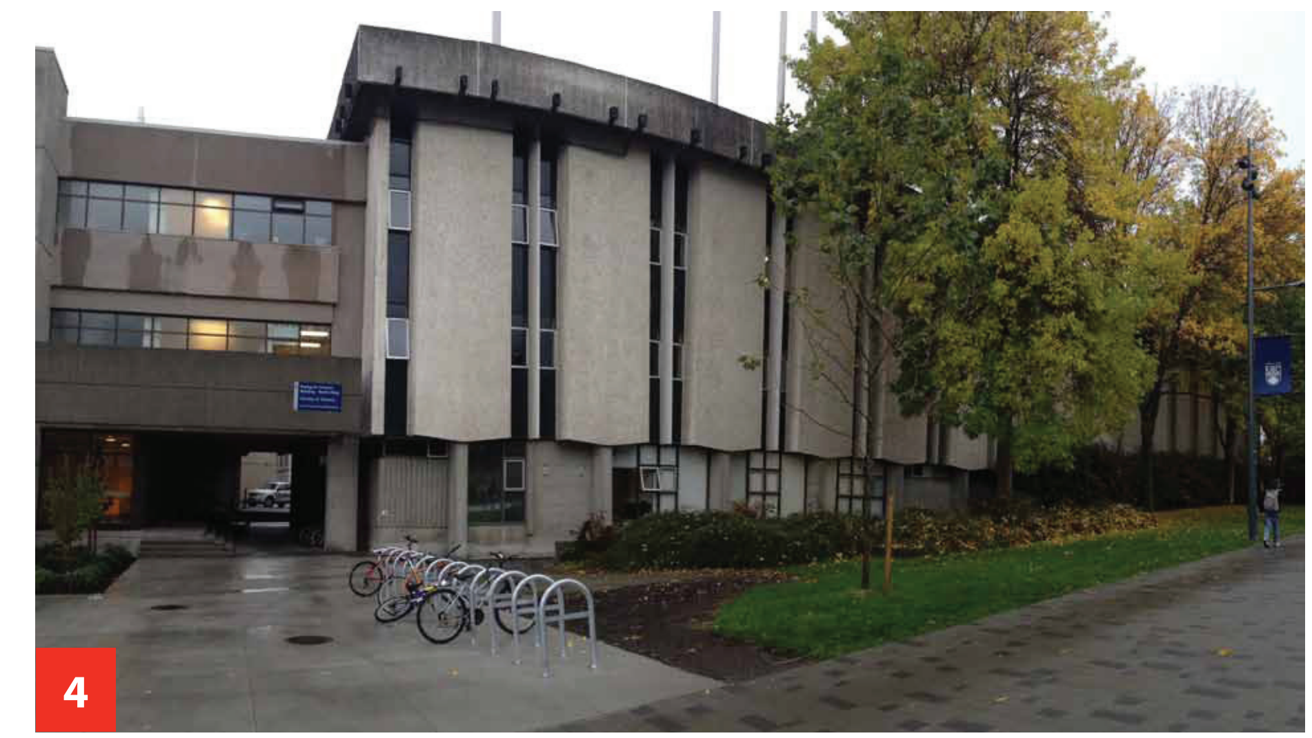
North east corner of North Wing
