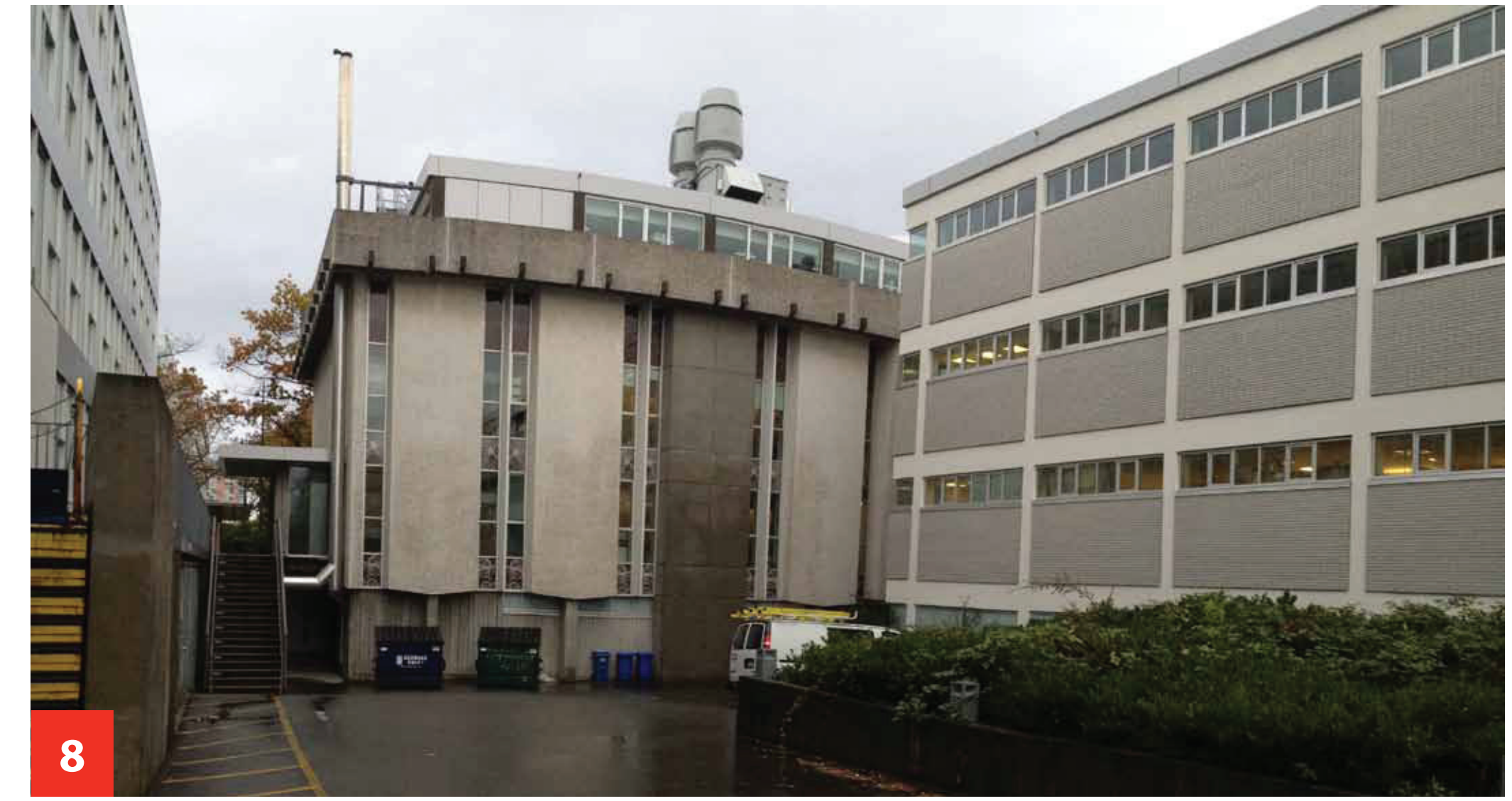
South west corner from service area
