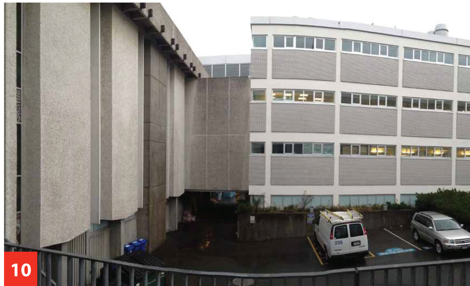
South west corner at service access to courtyard
