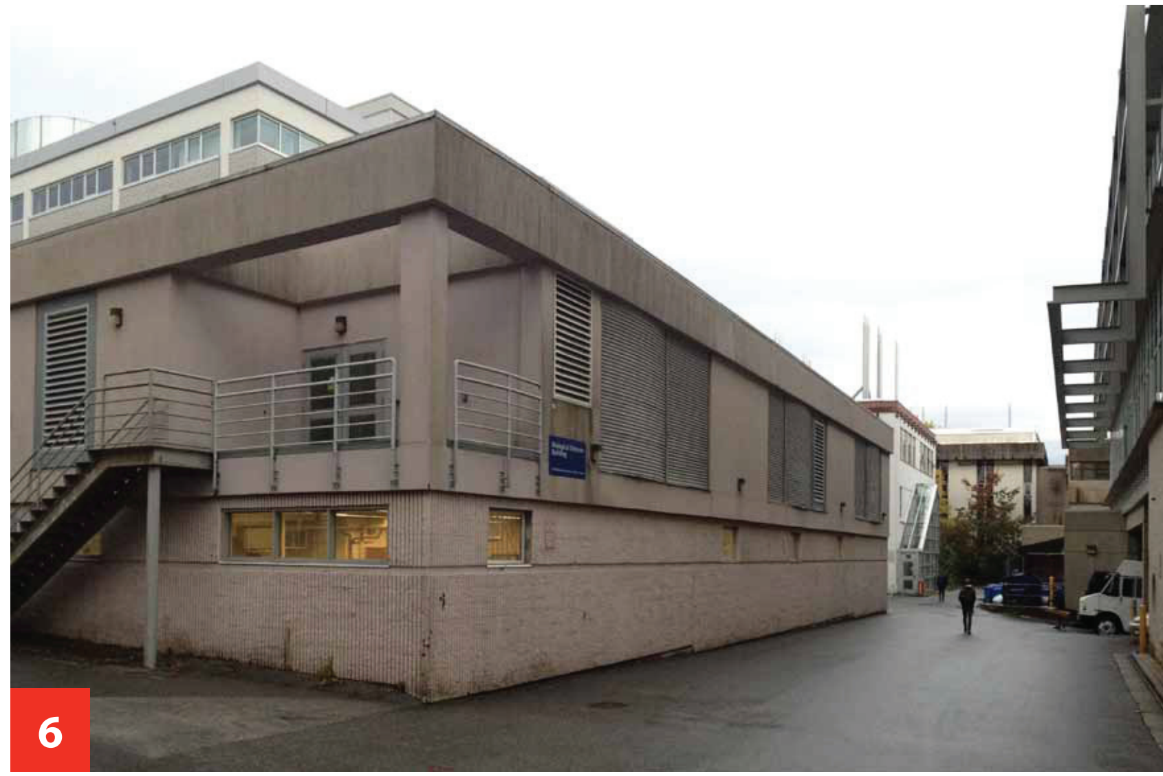
South east corner of south wing
