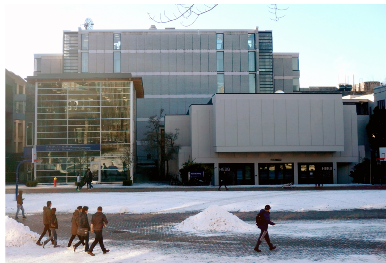
1 view of east elevation of Hebb tower and theatre
