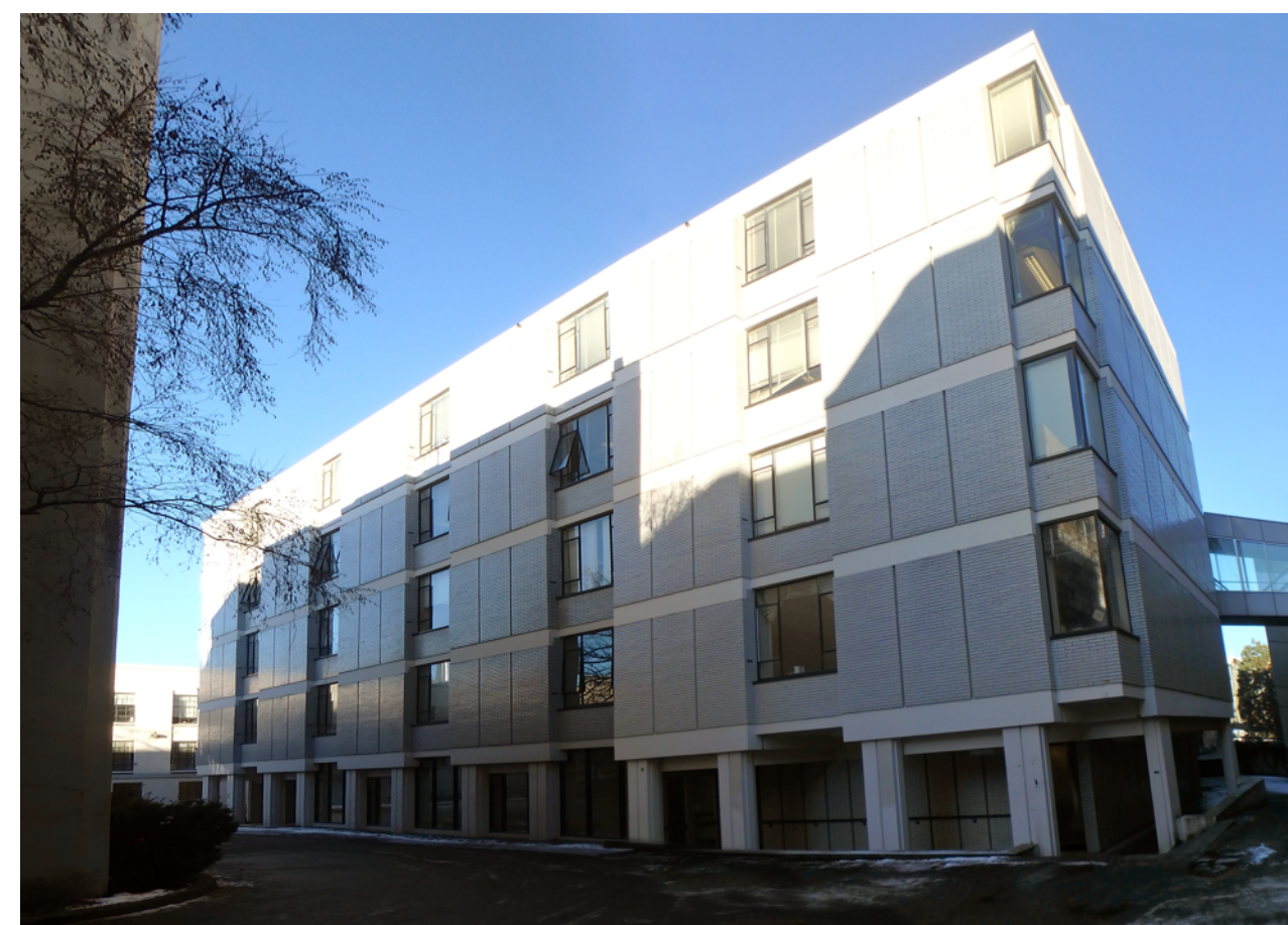
5 view of west and south elevations from south lane
