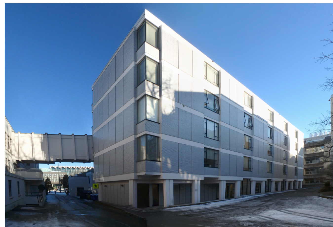
4 view of north and west elevations from Volkoff Lane
