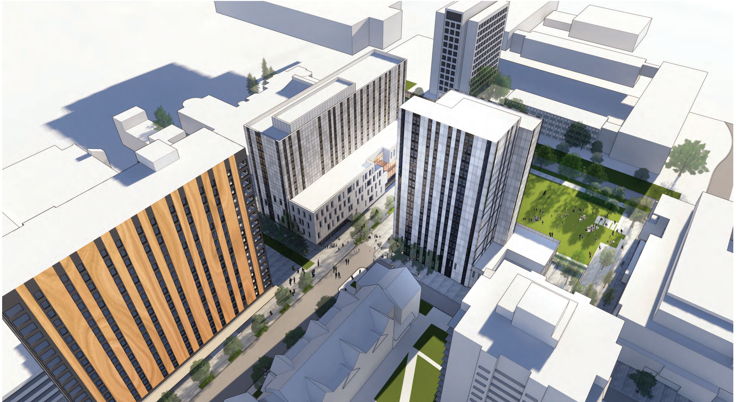
Aerial view to Southwest
