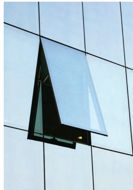
7. CURTAIN WALL GLAZING
