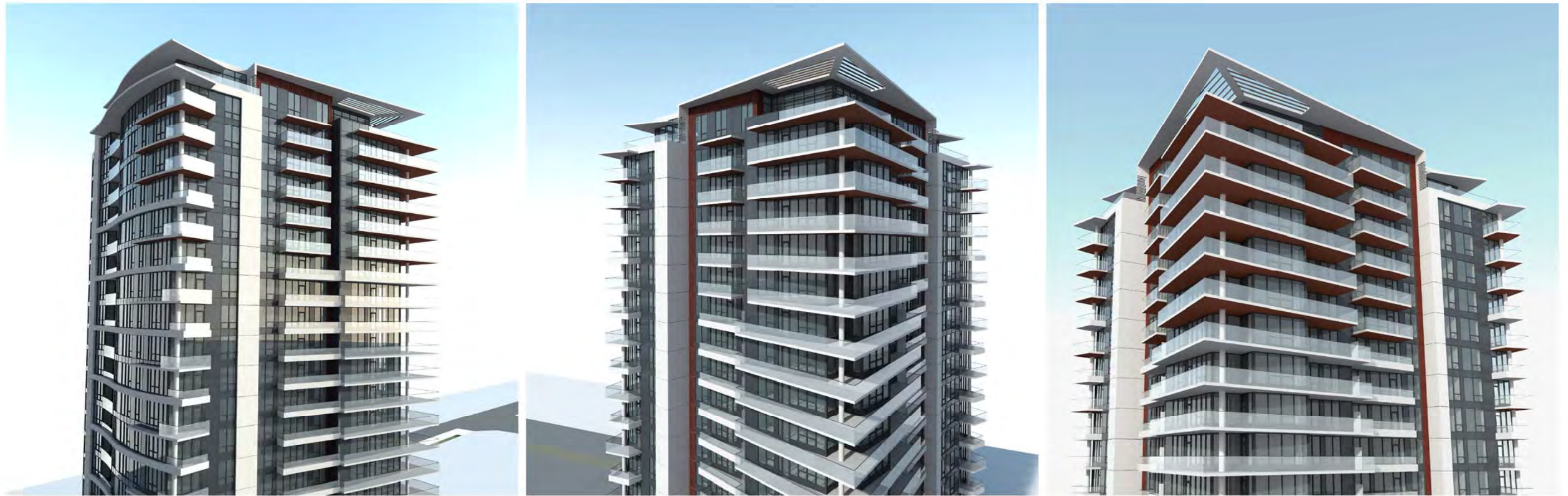
CLOSE-UP VIEWS OF TOWER ROOFLINES
