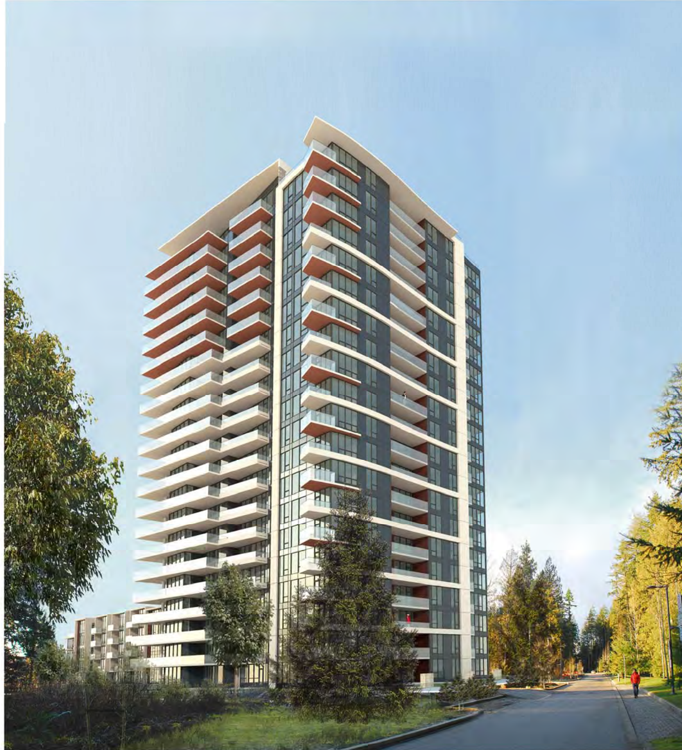
VIEW - SOUTHEAST ALONG BINNING ROAD
