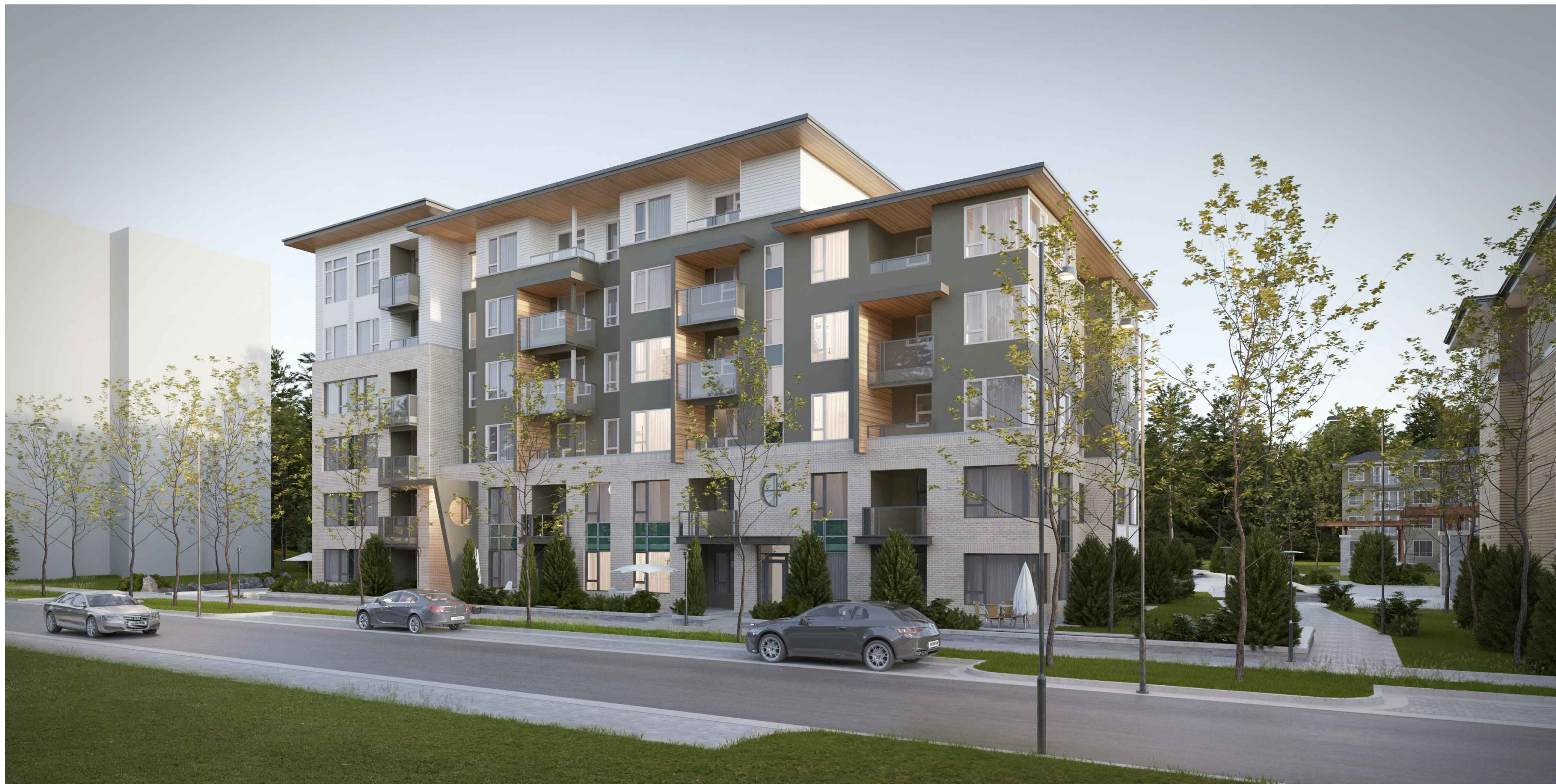
Ross Drive, South Building
