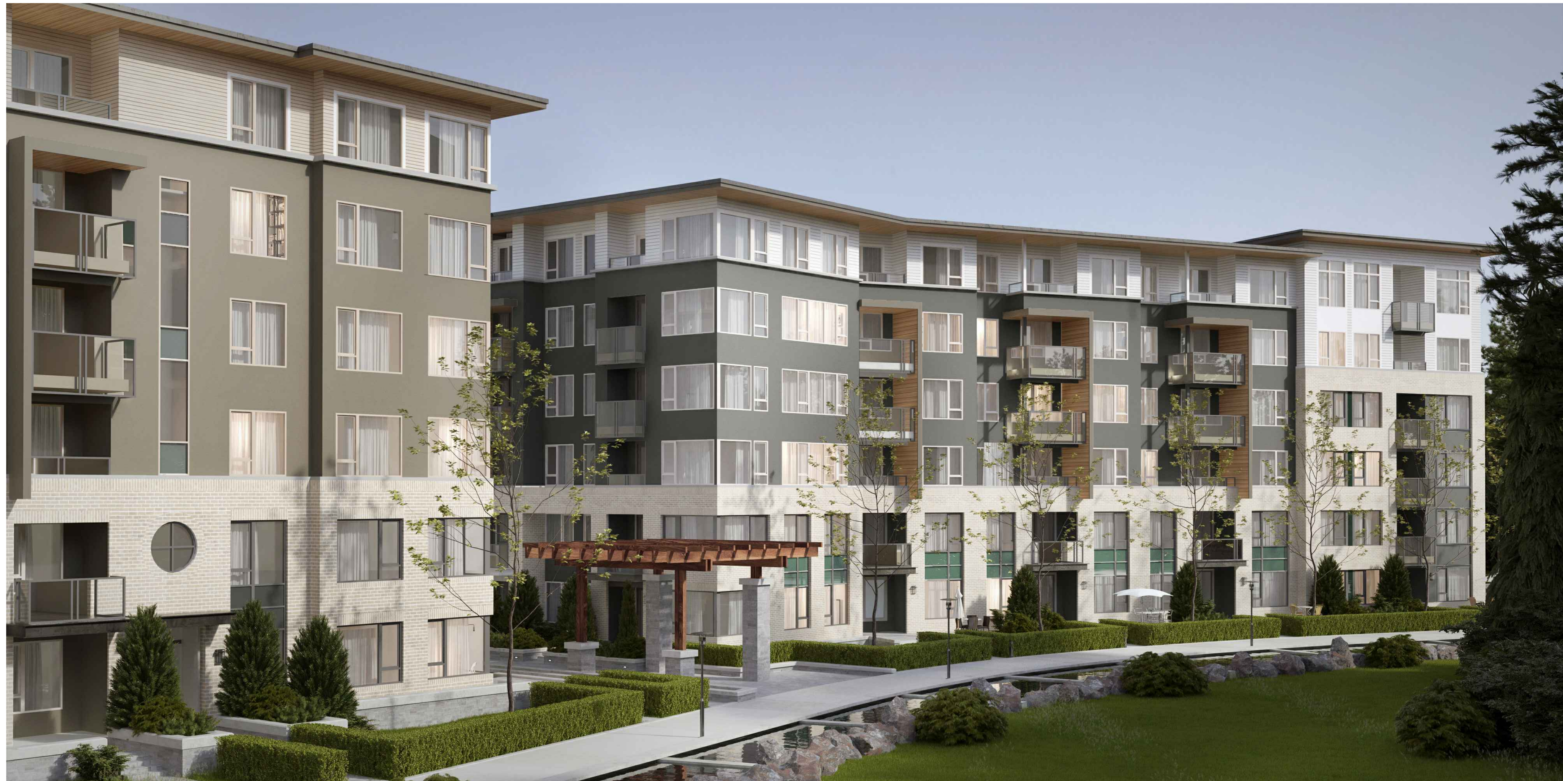
Pedestrian Mews, South Building
