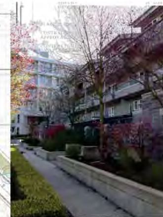
View From NE Corner of Building - Looking South
