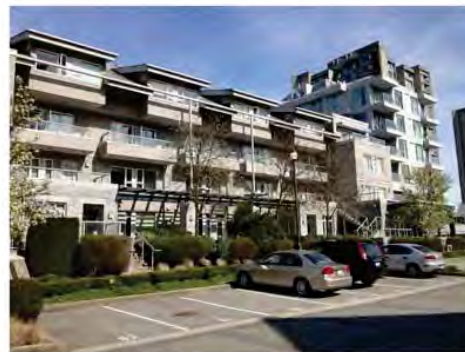
West Side of Building
