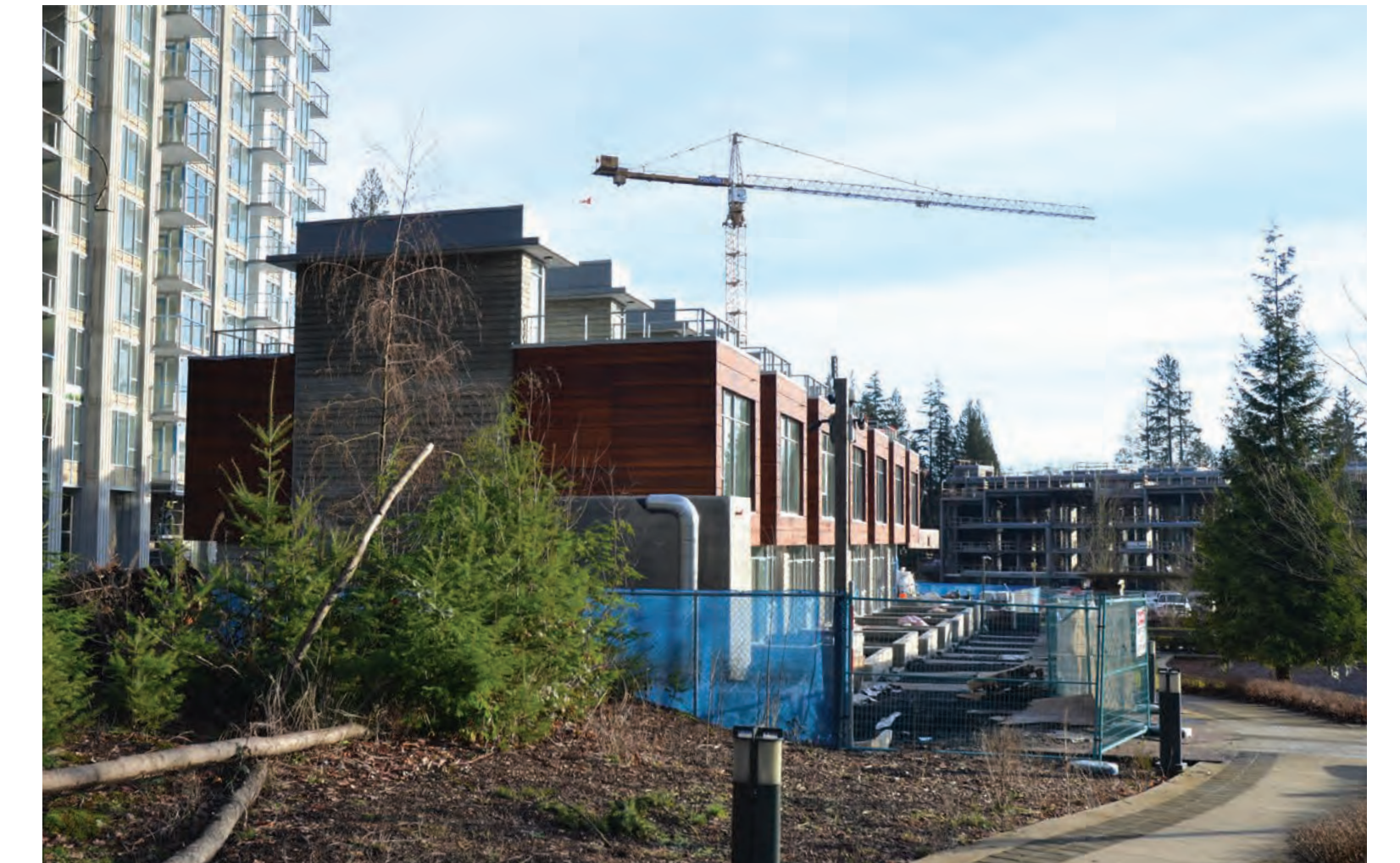
4 Binning and Laureates under construction
