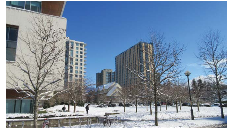
6. View towards Tall Wood from SW corner of Allard Hall
