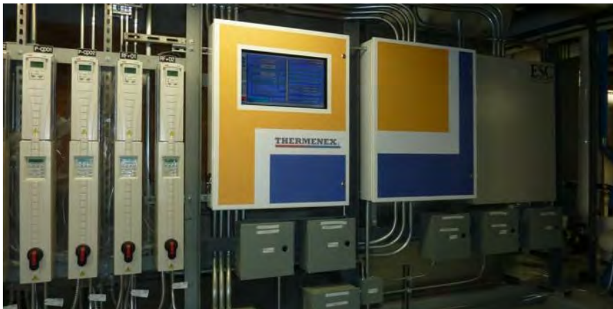
existing therменex heating and cooling system with monitoring and controls
