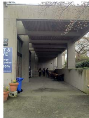
CORNER LOOKING WEST
