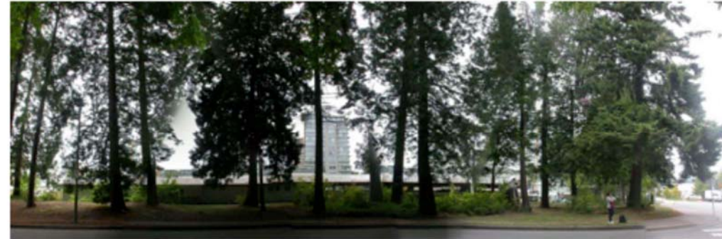
VIEW LOOKING NORTH FROM AGRONOMY ROAD (SOUTH ELEVATION)
