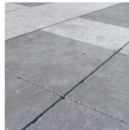
SAW-CUT CONCRETE
