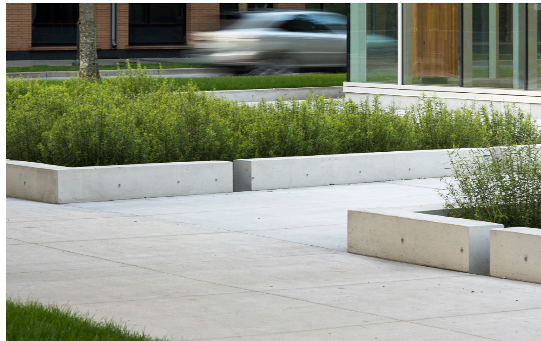
Cast Concrete Paving with Rectangular Planters
