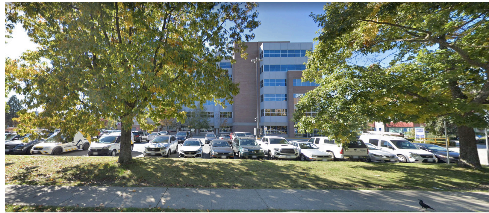
2 view of the site looking west from Health Sciences Mall
