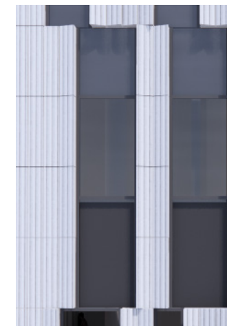
7. WINDOW WALL + SHADOW BOX; TINTED GLASS
