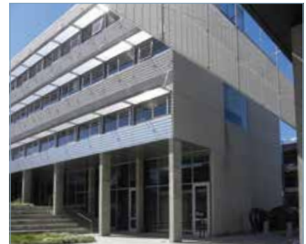
2.3.10.b.ii Buildings with extensive south exposure to consider strategies such as high performance glazing, shading devices or buffer spaces.
