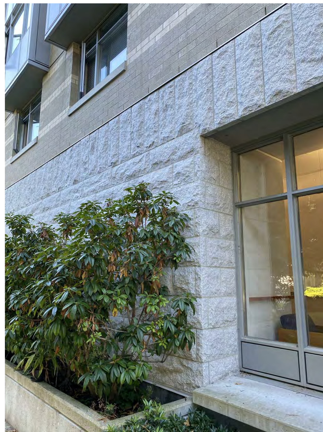
Fig.3 - Carey Hall (Existing 2005 Building) - Details at Interior Courtyard
