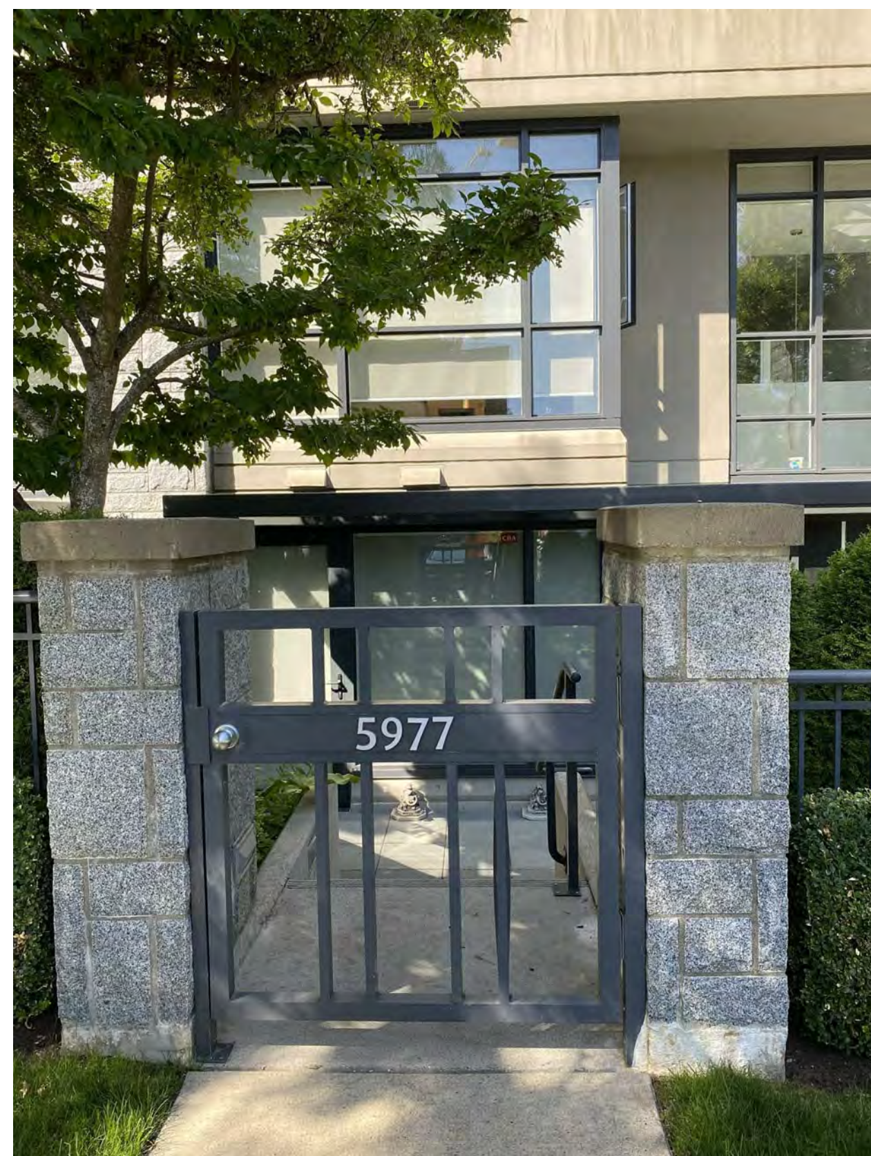
Fig.2 - 5977 Walter Gage Rd- Typical (Grey) Accent Colour, Quarried Stone, and Precast Concrete Caps/Sills
