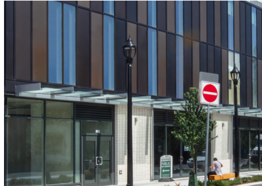
bronze anodized aluminum spandrel panels
