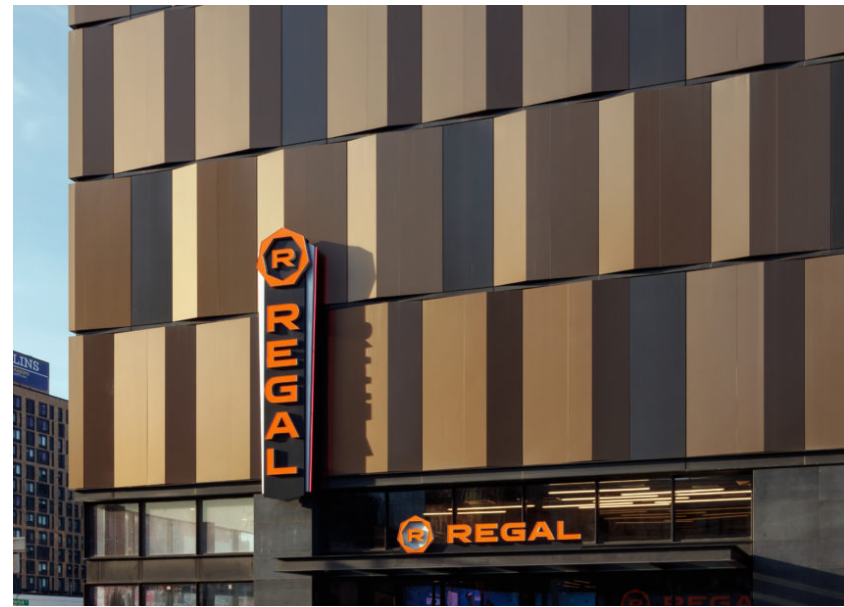
folded bronze aluminum composite spandrel panels
