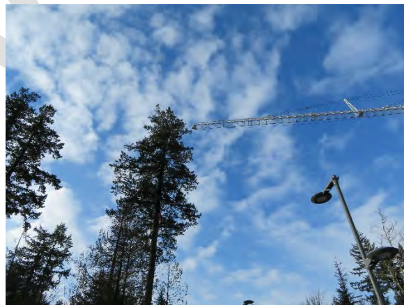
The crane on Lot 11 comes close to the edge of the furthest east tree in the vegetative buffer around the nest.
