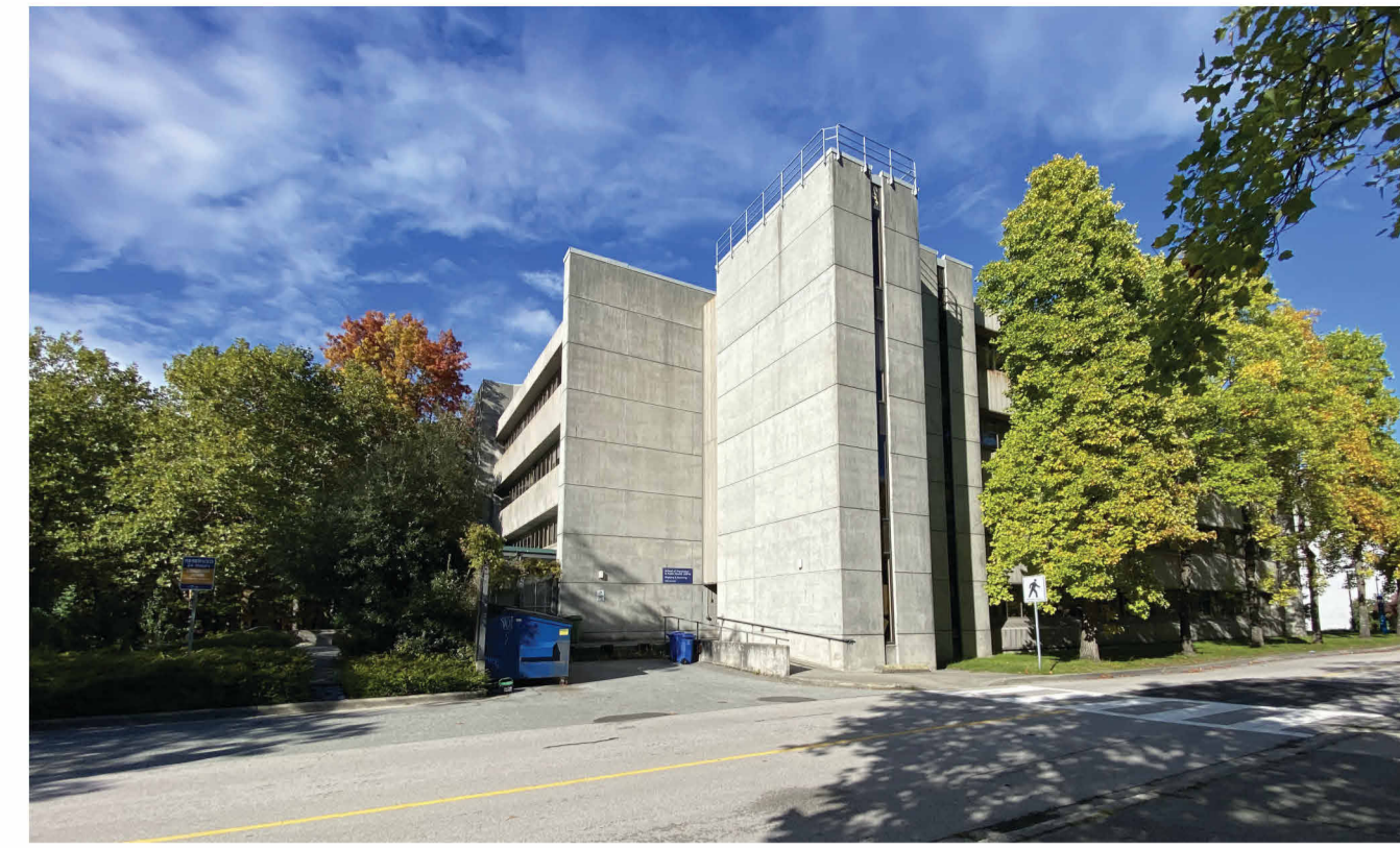
01 SCHOOL OF POPULATION AND PUBLIC HEALTH Loading Dock, looking North
