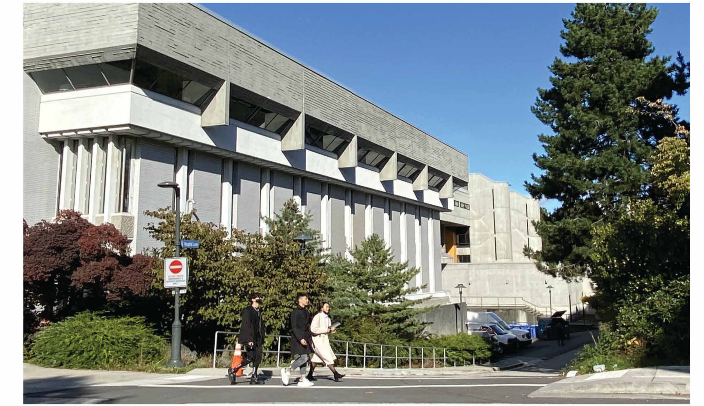
03 WOODWARD INSTRUCTIONAL RESOURCES CENTRE Southwest Corner, looking Northeast
