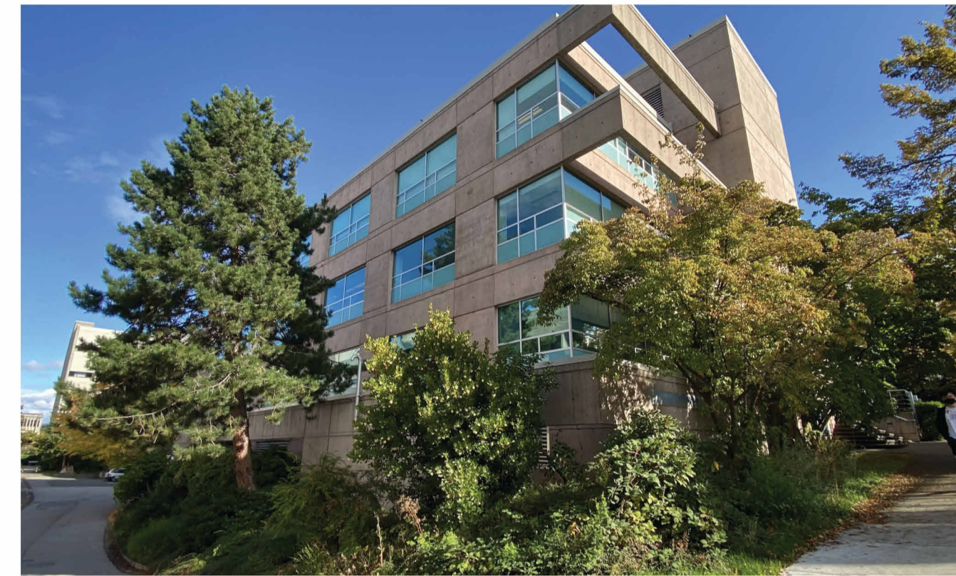
04 BIOMEDICAL RESEARCH CENTRE Northwest Corner, looking Southeast
