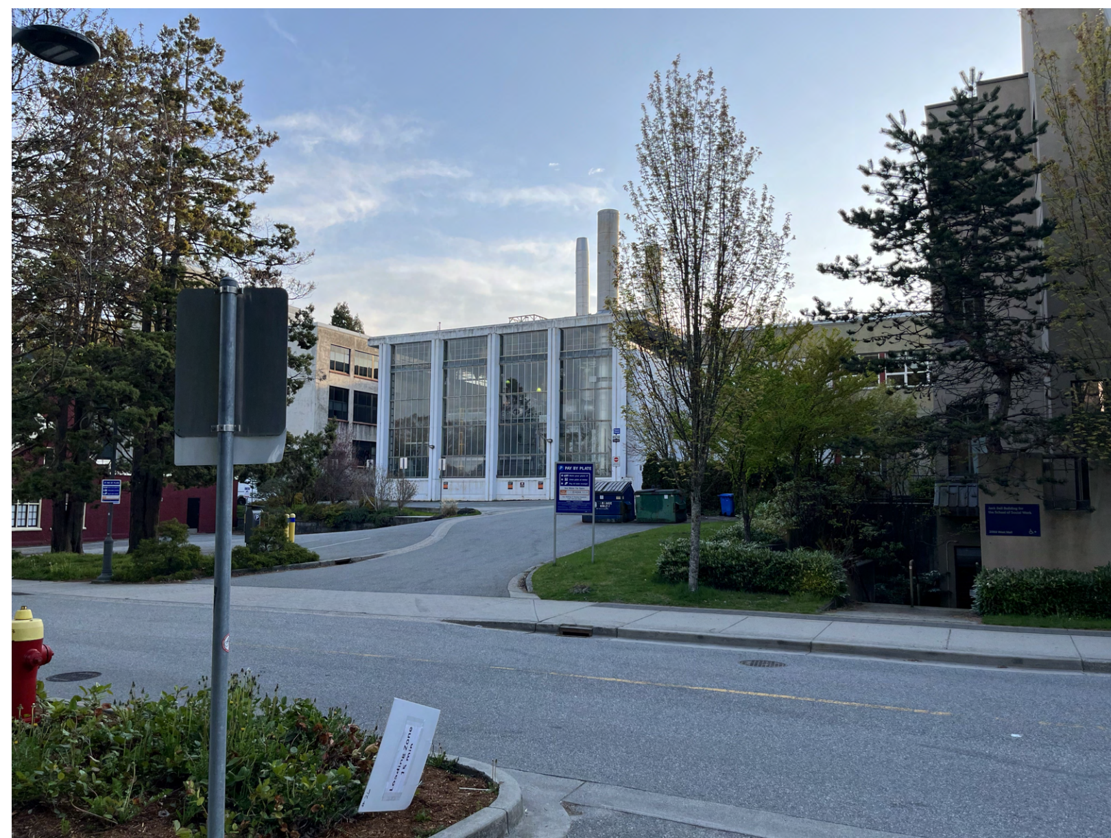
8 view of site looking north east from Ponderosa Commons
