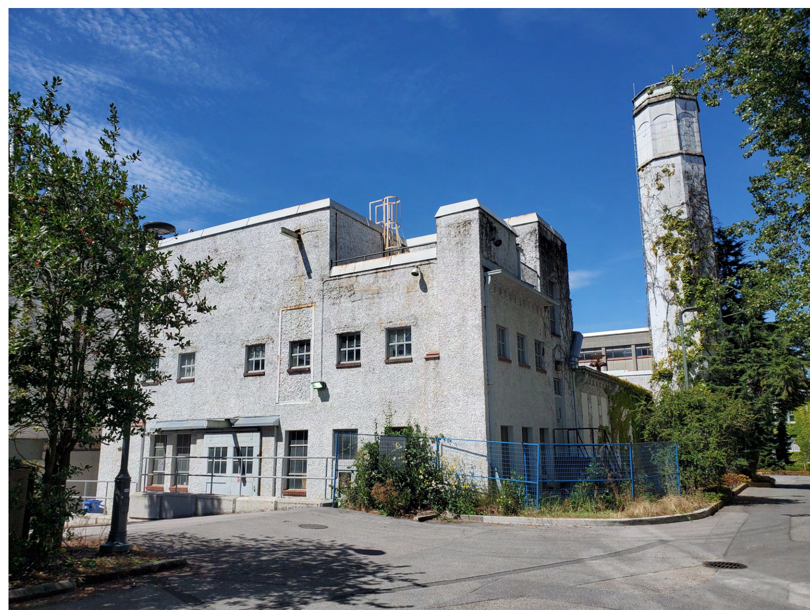
2 view of site looking north west from service lane
