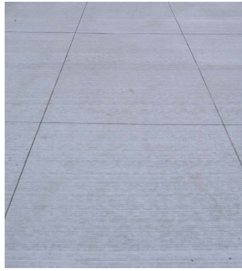
BROOM FINISHED CAST CONCRETE
