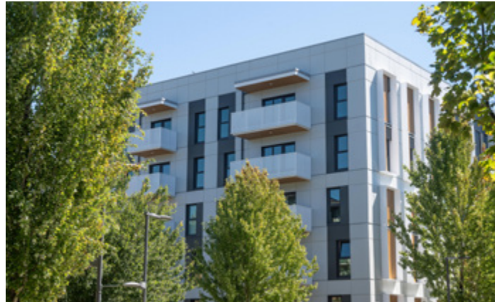
High performance neighbourhood housing (passive house) in Wesbrook Place Neighbourhood. (Photo Credit: Paul Joseph, UBC Brand & Marketing)
