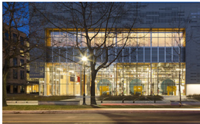
UBC Campus Energy Centre (Photo Credit: Ema Peter)
