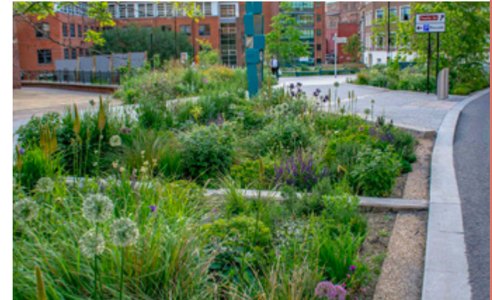
Rainwater garden integrated into street design. (Photo Credit: Nigel Dunnett)
