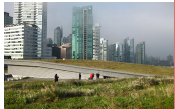
Rooftop pollinator garden enhances biodiversity and reduces urban heat islands. (Photo Credit: Daily Hive Vancouver)
