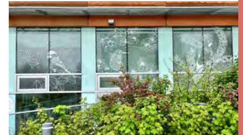
Bird-friendly building design on the windows of the CIRS building, integrating artwork from student Lora Zosia Moon, deters bird collisions. (Photo credit: Simone Levy)
