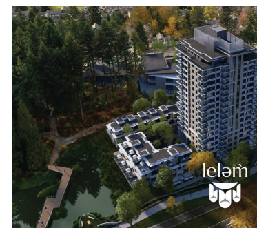
Create rich aquatic ecologies via green infrastructure that absorbs, cleans and transfers rainwater
