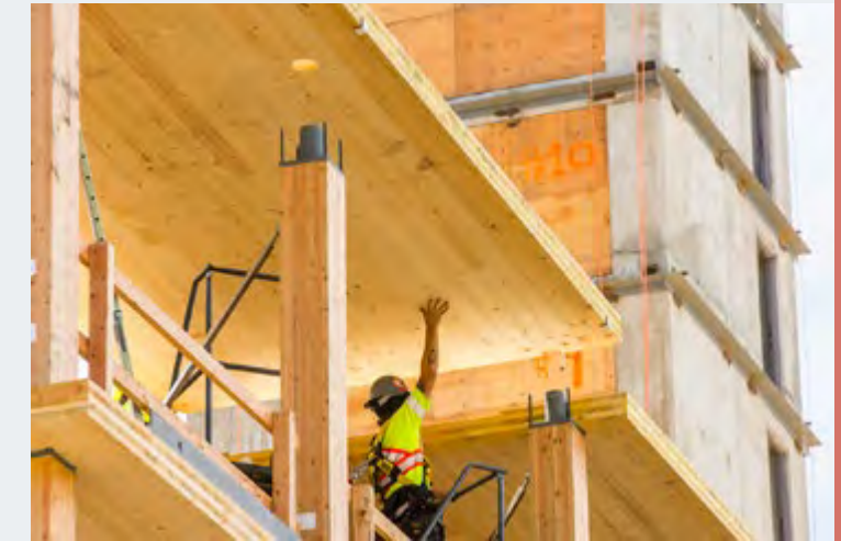
UBC was one of the first to test mass-timber hybrid construction in a high-rise building with Tallwood House, built in 2017. (Photo credit: KK Law)
