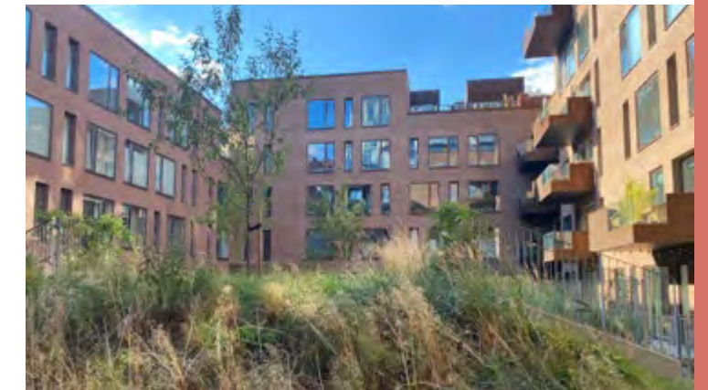
Residential courtyard with naturalized planting. (Photo credit: Gerry McGeough)
