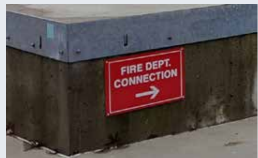
Directional FDC Sign at Earth and Ocean Sciences building -- new standard requires only the letters FDC.
