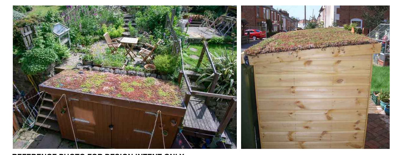
REFERENCE PHOTO FOR DESIGN INTENT ONLY - SEDUM ROOF
