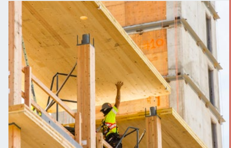
UBC was one of the first to test mass-timber hybrid construction in a high-rise building with Tallwood House, built in 2017. (Photo credit: KK Law)
