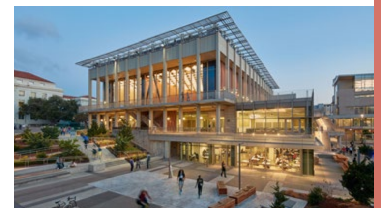
Lower floors provide social and community spaces that activate the public realm. (Photo credit: Bruce Damonte)
