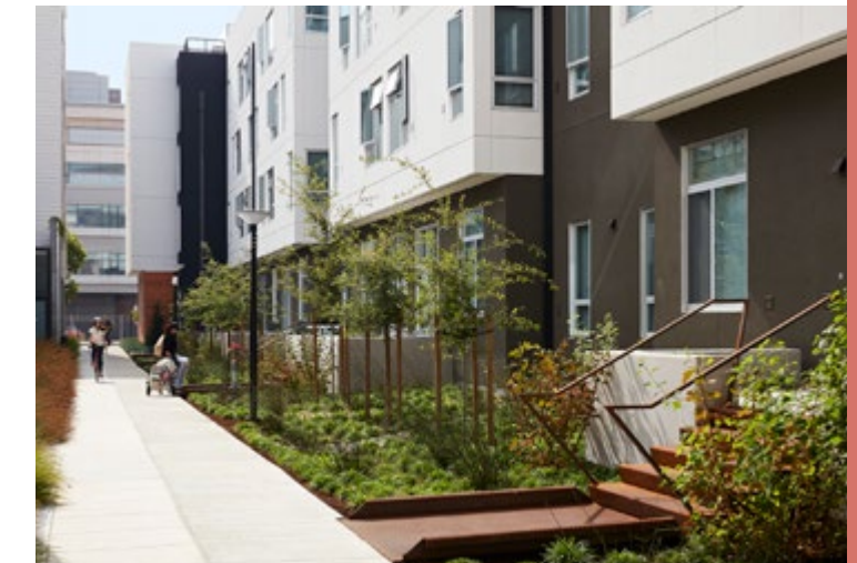
Mid-rise scale housing with front doors onto the public realm. (Photo Credit: Mariko Reed)
