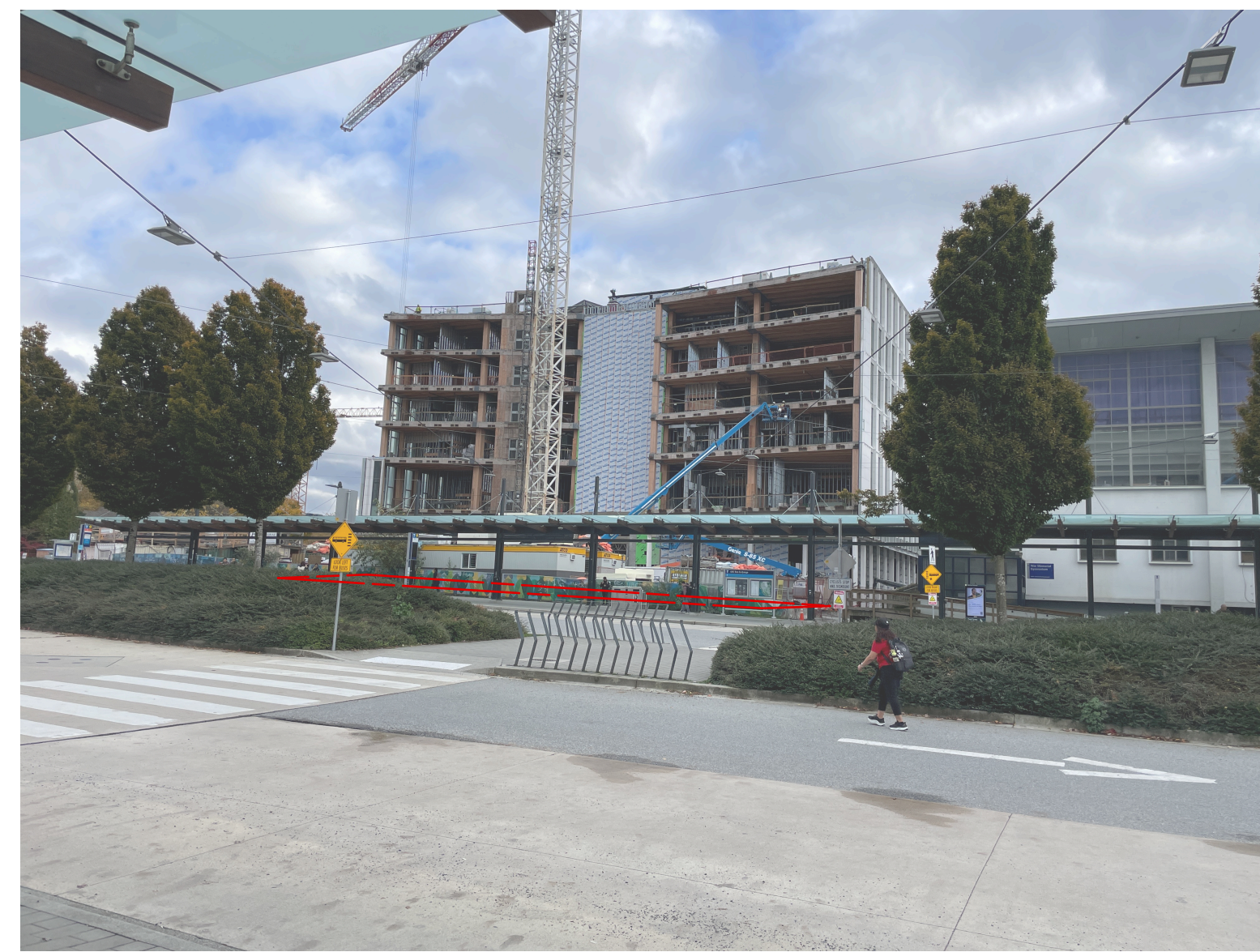
4 view of the site looking southeast from the bus loop
