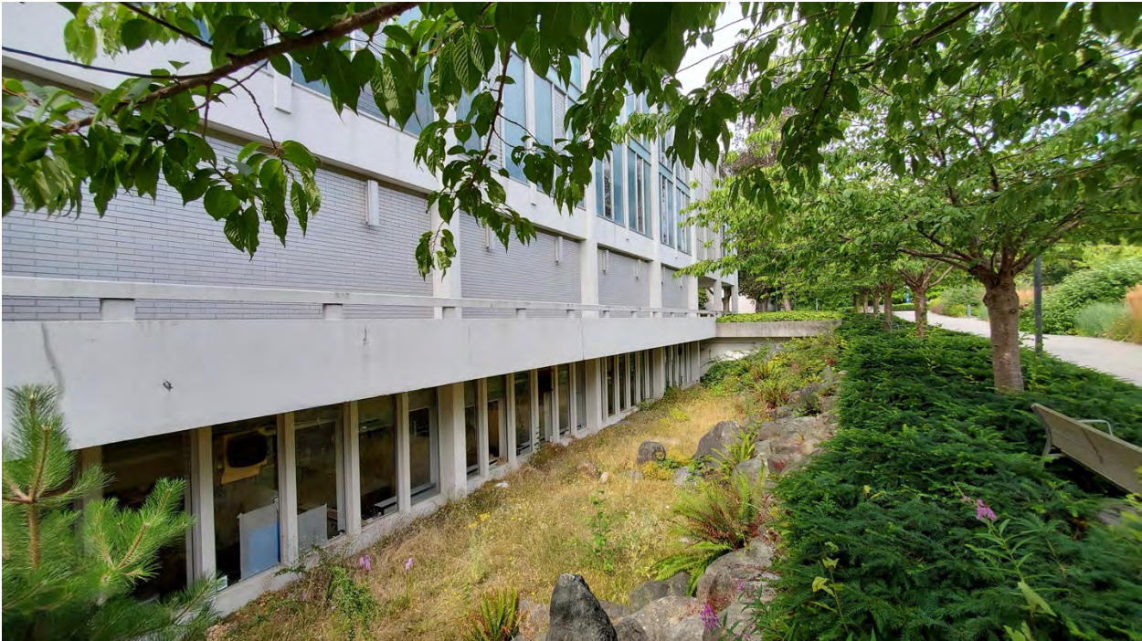
Sunken level along south elevation
