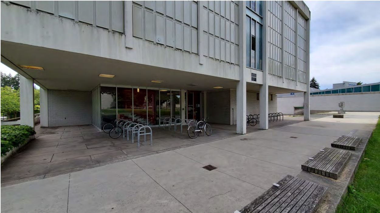
Entrance on east elevation
