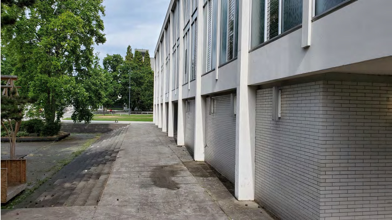
Pilasters and brick
