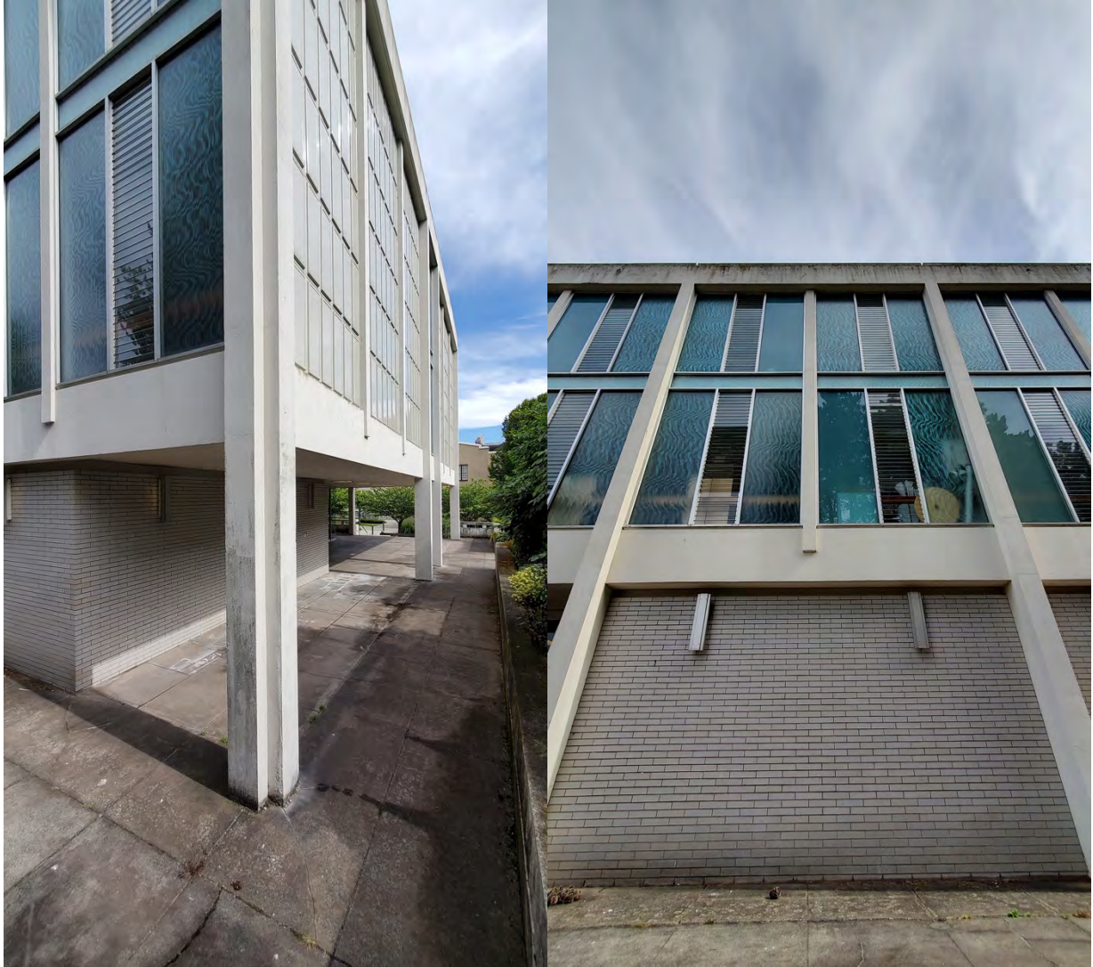
Columns and cladding
