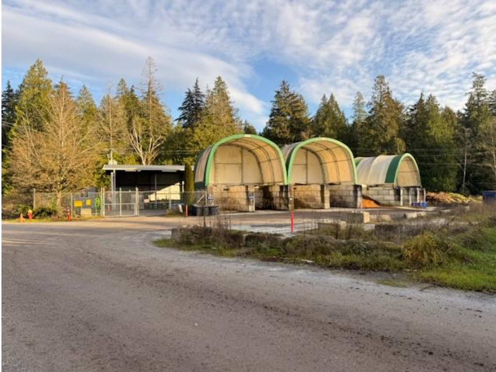
Photo 7: Onsite sorting area for recycling.
